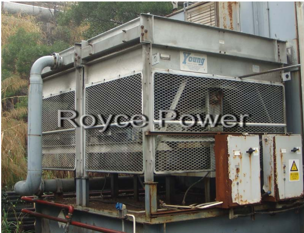
Engine Jacket Water & Auxiliary Radiator [Young]
